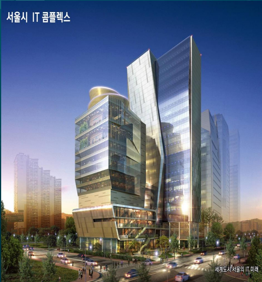
Seoul Metropolitan IT complex cloud computing data center.
