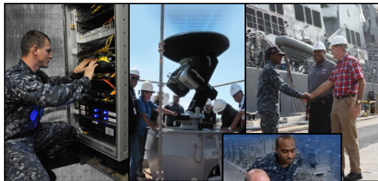
Production, Installation In-Service Support
