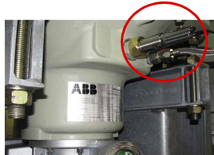
Humidity sensor on a GIS, Vaisala
